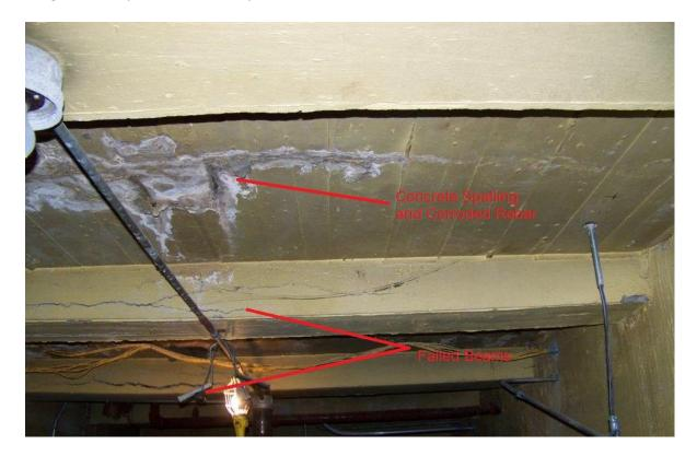
It was evident that, over time, water has migrated into the concrete cracks and corroded the reinforcing within. Eventually the reinforcement corrosion expanded and increased the cracks widths to a degree that repair is not practical.
